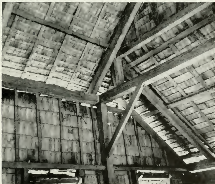
FIG. 18. Upper: A new item in village architecture. Two-story house under construction. Lower: Interior of a thatch house, showing construction of roof and wall.
