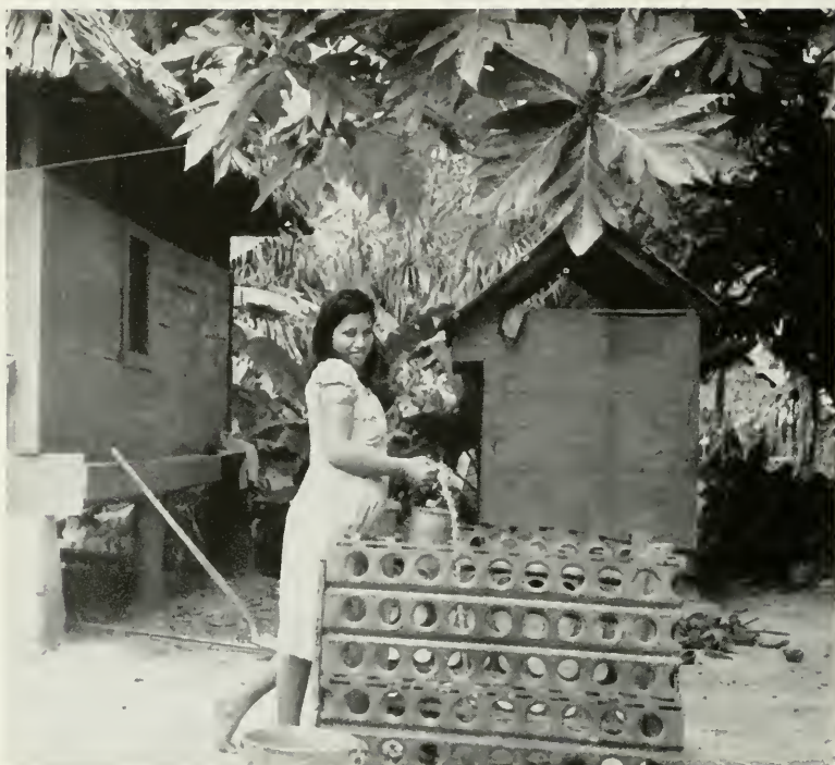
FIG. 25. Drawing water from a shallow well. The small house in the background is a bath-house. The grating around the well is Marston matting salvaged from the Navy base.
