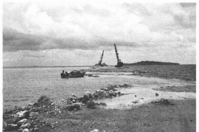
Silt and sediment produced from uncontrolled dredging and poor causeway construction have resulted in the elimination of marine life in many lagoon areas throughout Micronesia.
