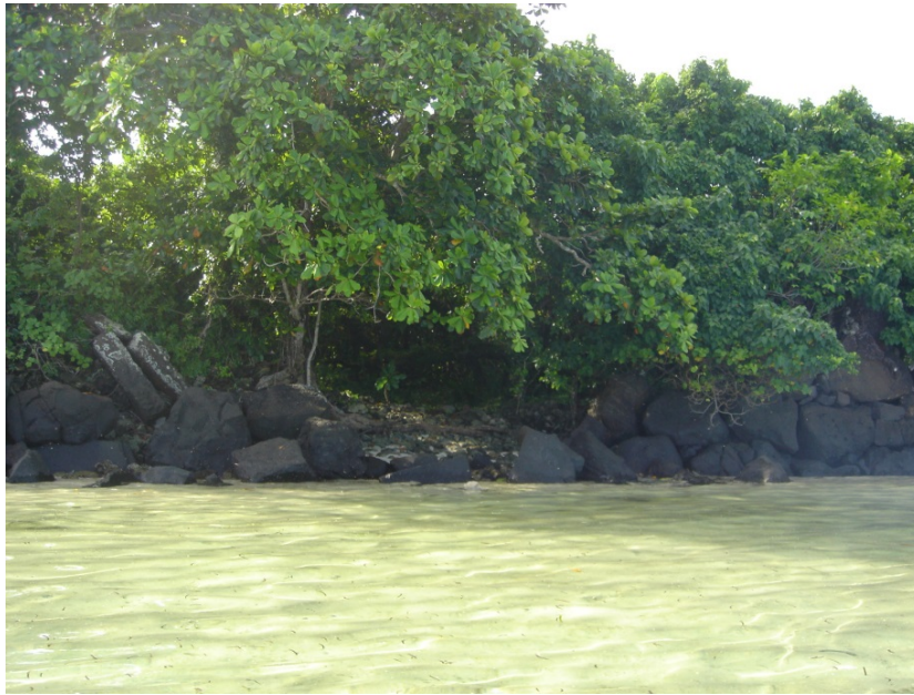
Figure V-4. A disturbed area along E seawall of Nan Madol (Angeir-Sapwuhtik B) This reflects a combination of wave damage, remodeling, and settling of architectural fill.
