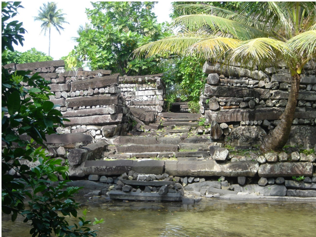
Figure III-6. Nan Douwas islet exemplifies header-stretcher construction at Nan Madol.
