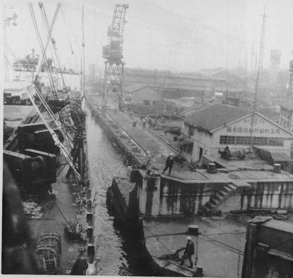
Above: The Gunners Knot moves into the dry dock at Osaka, Japan. Below: As the water is emptied from the basin, shores are put into place for support.
