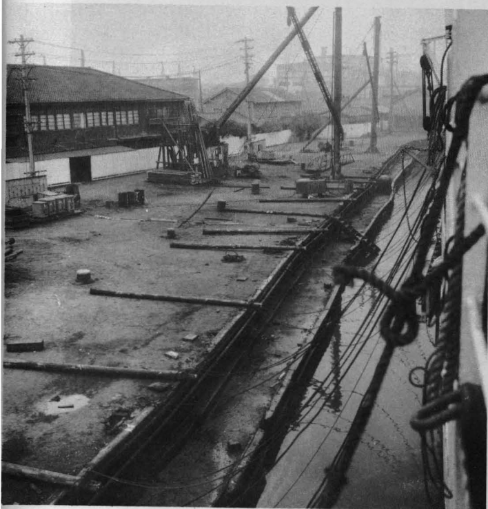
Above: The Gunners Knot moves into the dry dock at Osaka, Japan. Below: As the water is emptied from the basin, shores are put into place for support.
