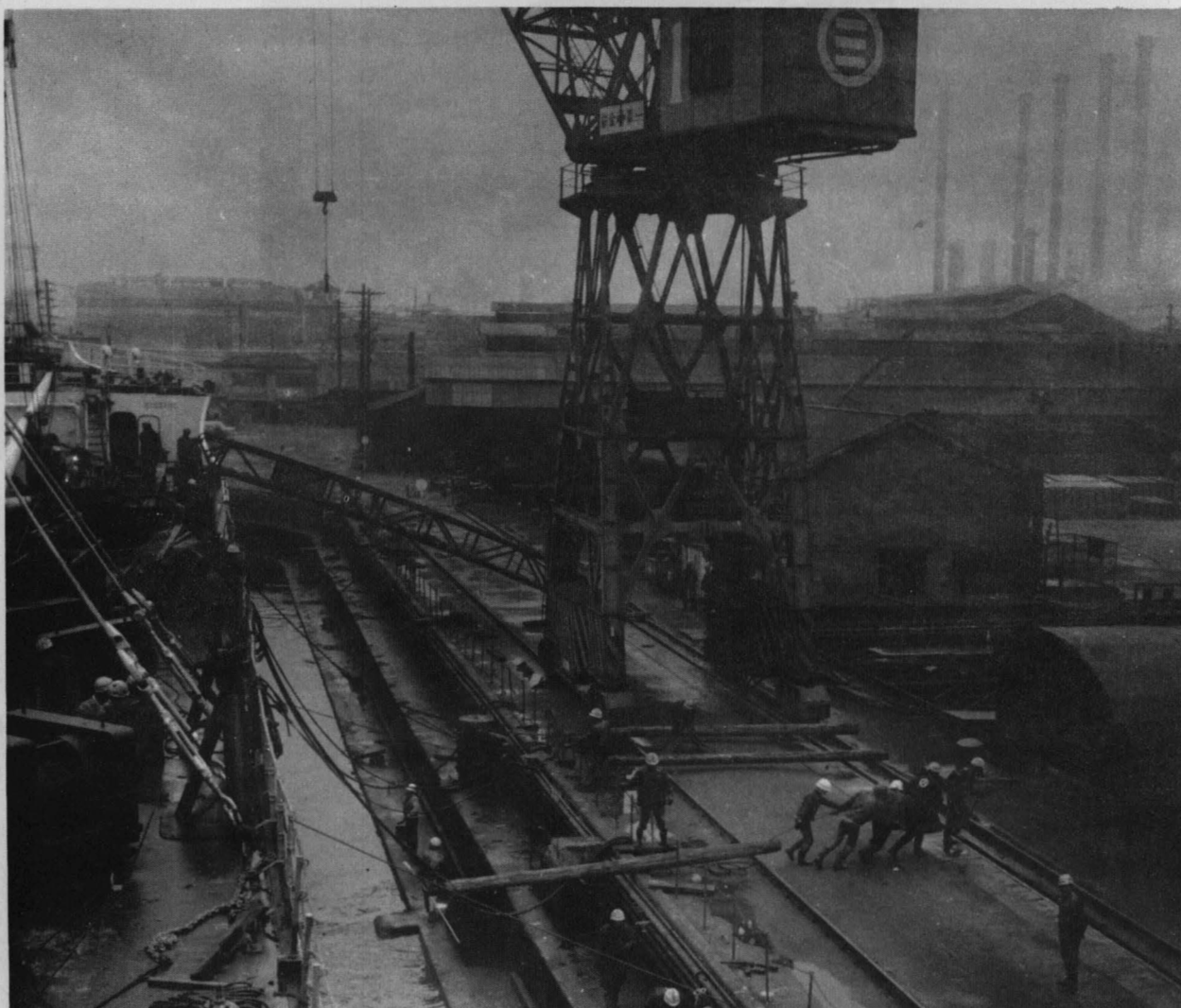
The shores are removed and the Gunnars Knot is now ready for final inspection and then will go to sea.
