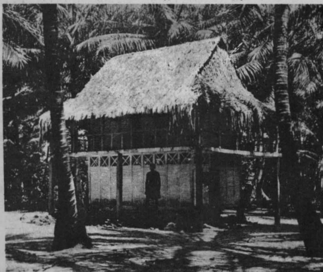
A two-story dwelling house. Three large center posts usually supported the central beam of dwelling houses, while along each side were three of four house posts, commonly set six feet apart. The houses were thatched with the leaves of the ivory nut or coconut. Dwelling houses of the early eighteen hundreds appear to have been very similar.
