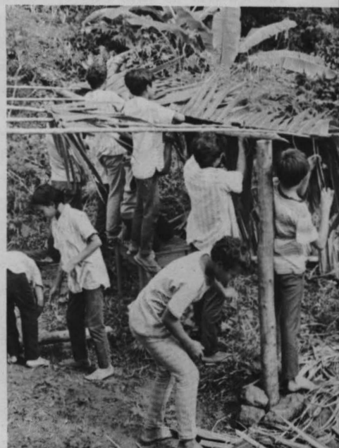
Palm branches, mangrove posts, coconut fiber twine, and the limitless energy of seventh and eighth grade boys combine to construct a new cookhouse at Nan Uh school. One of two surviving schools built by the Japanese, Nan Uh was designed for three grades. Before Saladak opened in 1968, Nan Uh was hosting eight grades.
