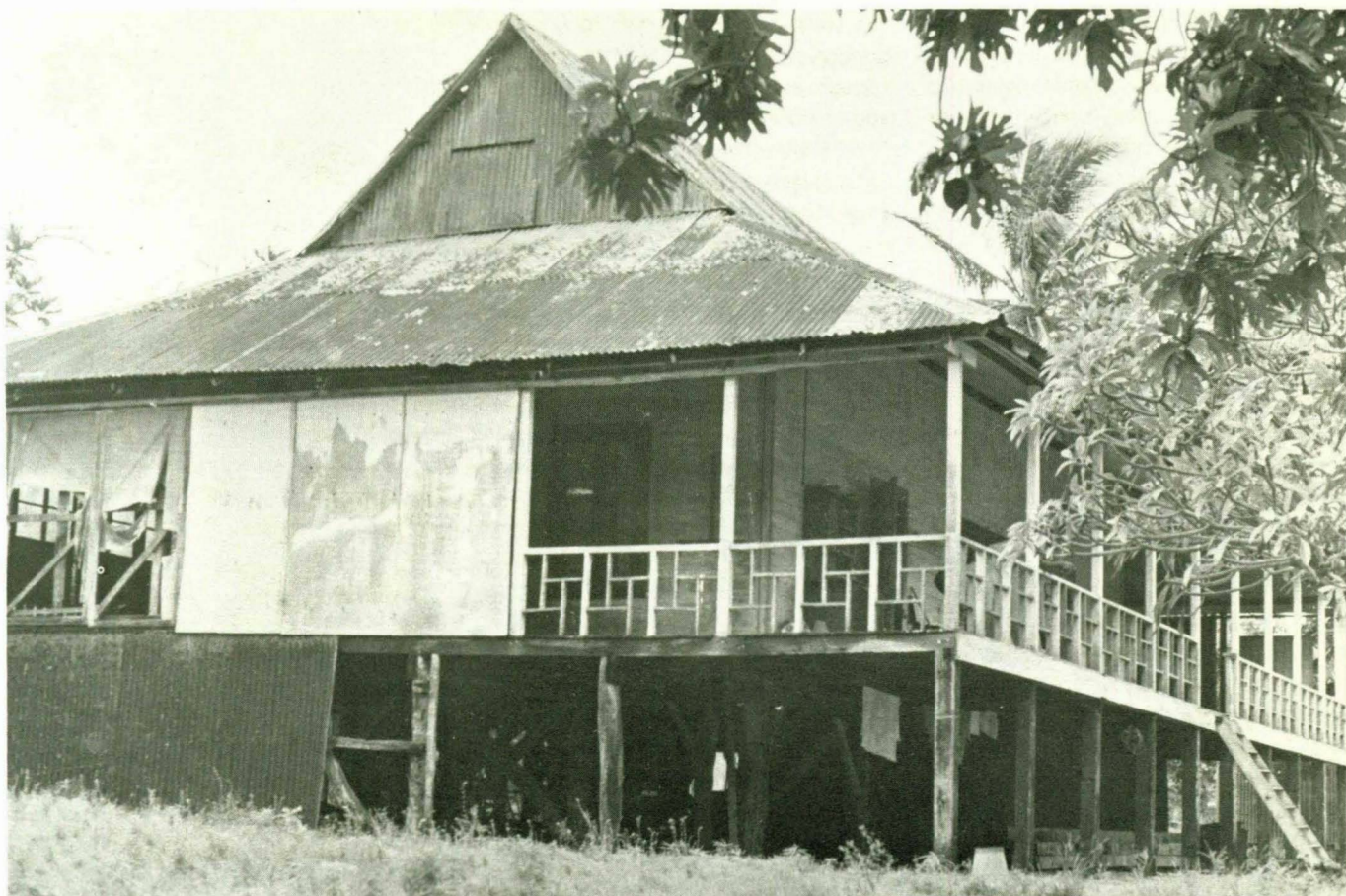
View of the mansion after most of the supports have been replaced but before the installation of the new roof. Although the mansion has been "stabilized, there is still much left to be done.
