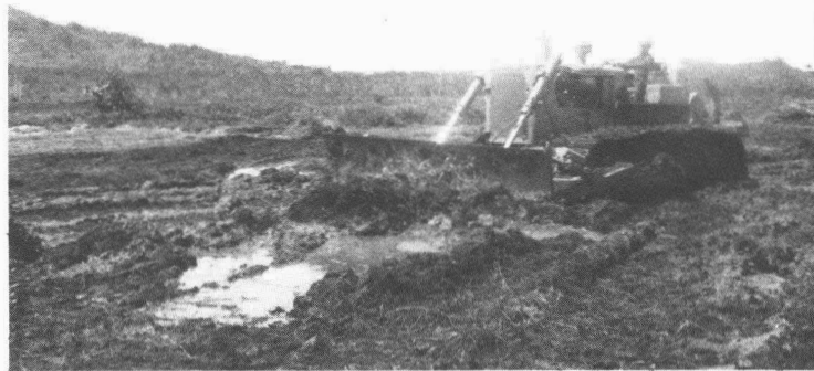
Special wide-track bulldozers grade rice paddies on Ponape.
