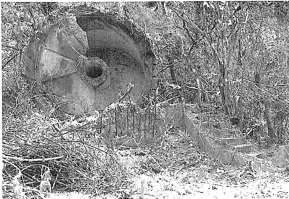
Plate 3. Base of the toppled lighthouse tower, foundation, and northern staircase.
