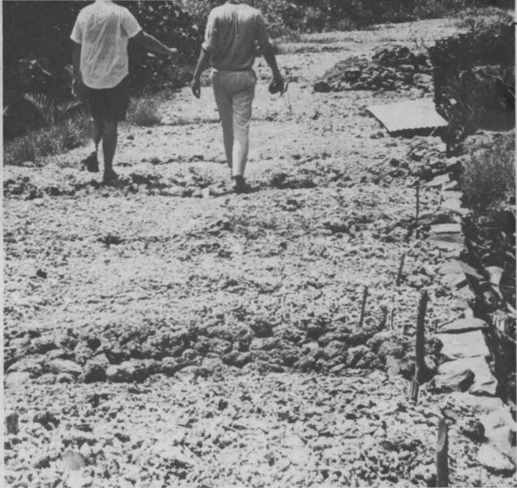
Indelible trademarks of the PTB's approach to road construction are these side-long hammocks of coral. The coral must be hauled out of the sea, brought to land in barges, dragged through mangrove swamps up to the road site.
