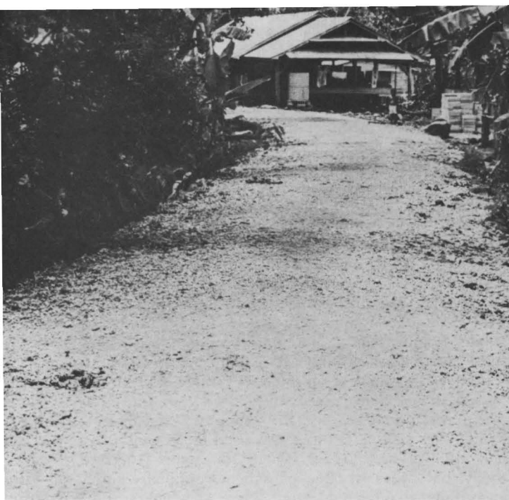
Here are the results: block coral covered with finger coral, levelled, packed and rolled. Fully wide enough for two jeeps to pass, the Sokehs road is as ambitious a reconstruction project as the Ponapeans have seen in decades.
