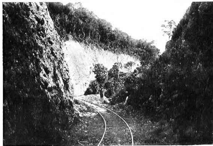
(4) Railway construction work in Saipan.
