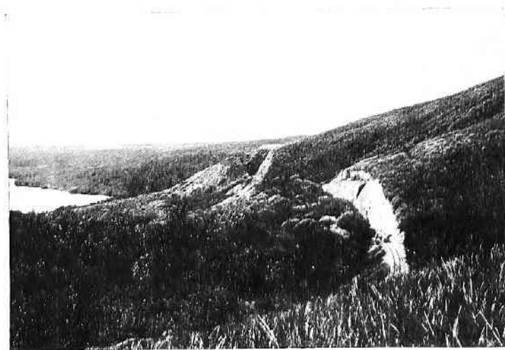
(3) Railway construction work in Saipan.
