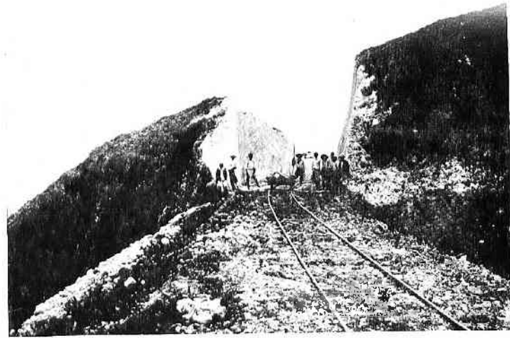
(2) Railway construction work in Saipan.
