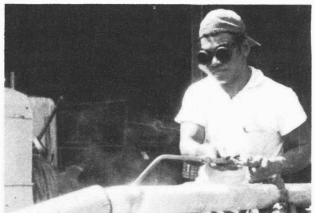
YAPESE WELDER FOREMAN Silvester Alfonso welds pipe in preparation for installation of additional generator unit, Yap power plant.
