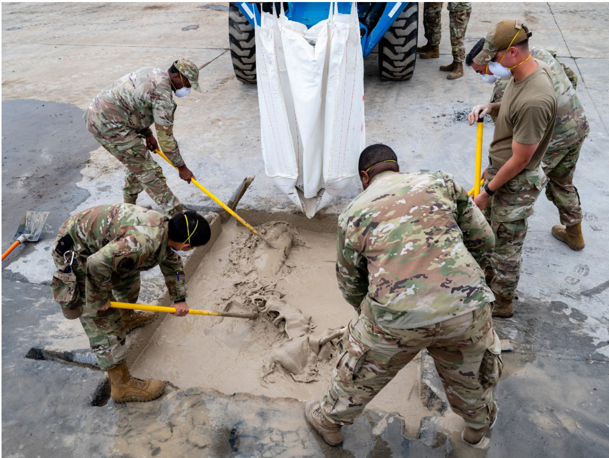
IMAGE 1. The 374th Civil Engineer Squadron Repair a Crater with Flowable-Fill During a RADR Exercise at Yakota Air Base, Japan, August 22, 2024.
