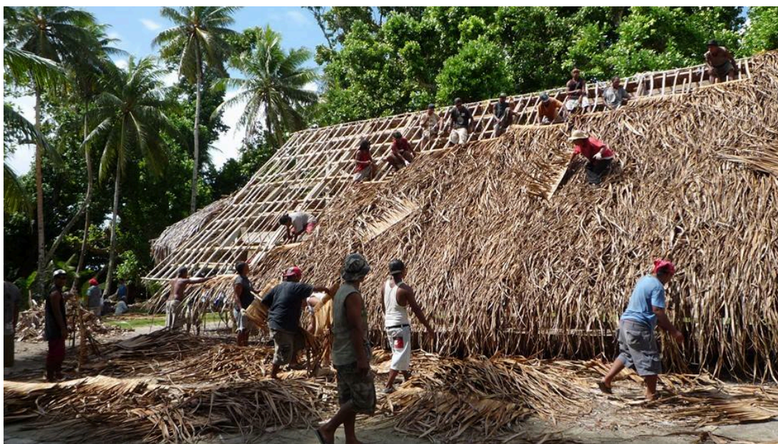
Figure 19: People of Rewow village, in 2014, on Lekinioch work together to replace pandanus sheets on foeng the ainang faal of Sopunpi . The principle of alilis fengen is noted here.
