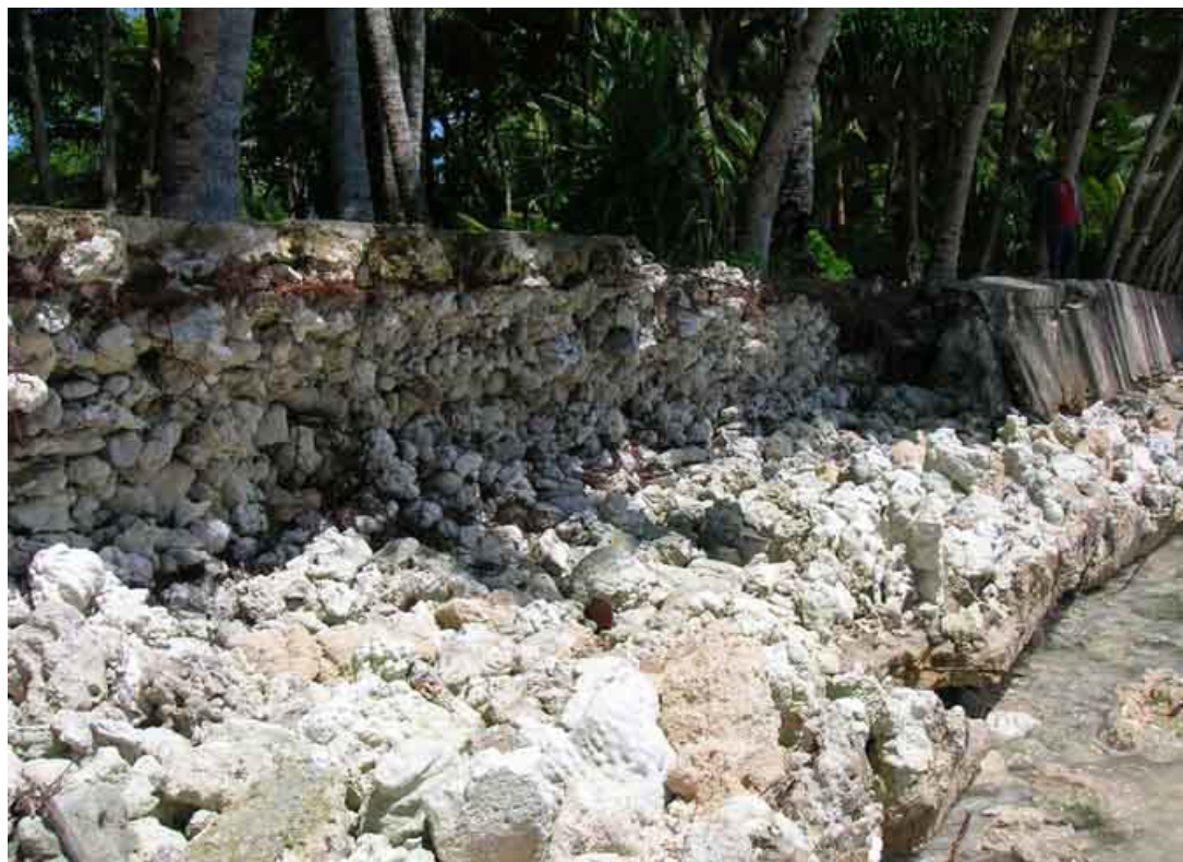
Figure 17: Old style sea wall on the island of Lukunor constructed in the 1970s. It fell apart shortly after its construction due to lack of the elders input into the project.
