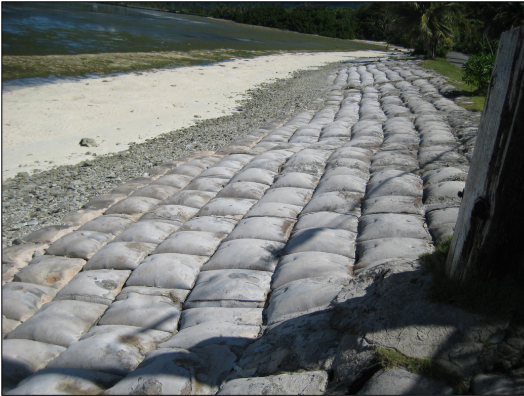
Figure 18: New sea wall design in Kosrae to prevent beach erosion. Picture taken by Zag Puas on June 23, 2012.
